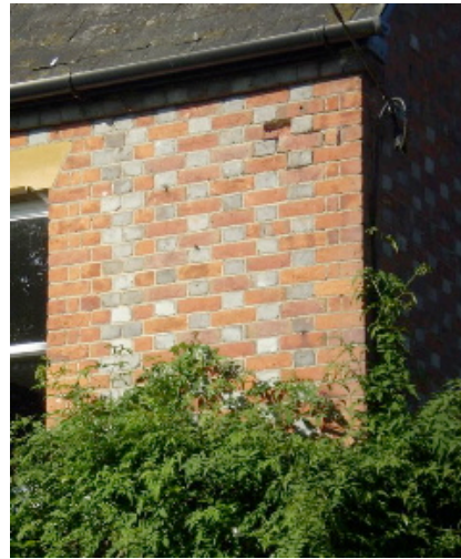
Flemish Bond brickwork
