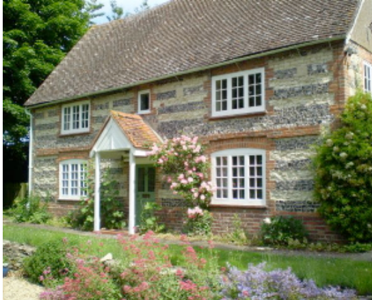
'The Wellsprings', built 1689 in a characteristic local style of banded chalk clunch, flint and brick
